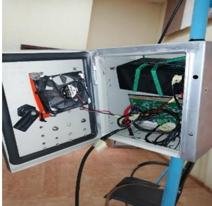
Figure 6. Transceiver installation in the casing
