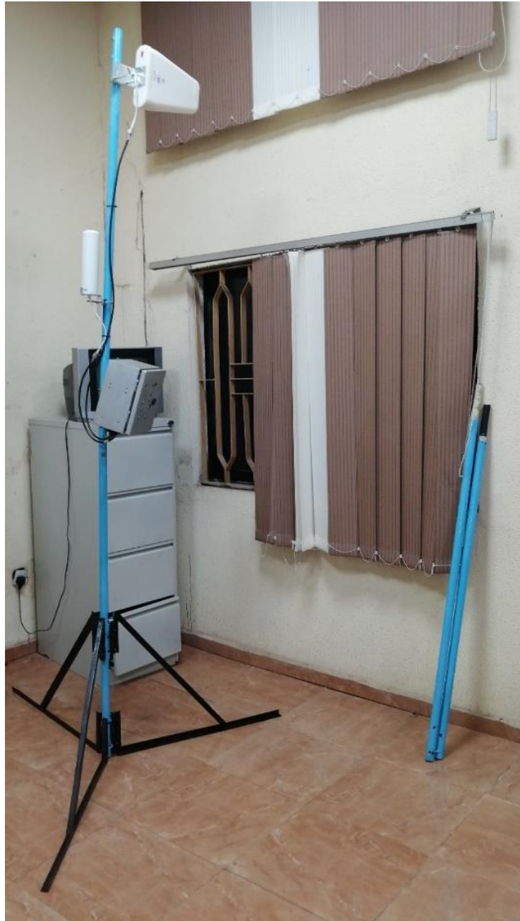
Figure 14. Complete Transceiver Installation Package
